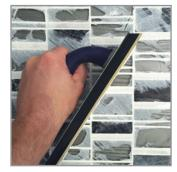
Remove excess grout through successive diagonal passes using the edge of the rubber float held at a sharp 90° angle.
