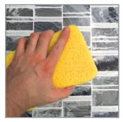
Allow grout to harden for about 20 to 30 minutes. Using a slightly damped cellulose sponge, losen up all excess grout over the tile with a circular motion. Do not add water before all is well loosened up.
