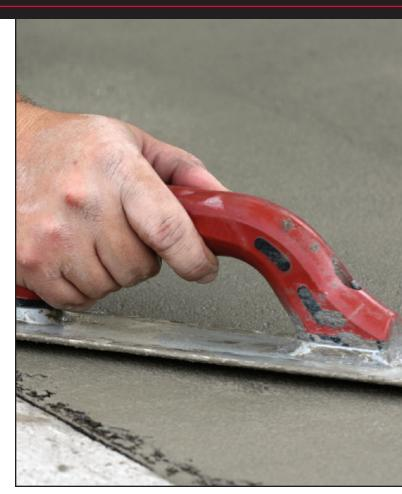
Surfaces must be clean and free of dust, oil, grease, paint, tar, wax, curing agent, form release agent or any deleterious substance and debris which may prevent or reduce adhesion. Mechanical removal of poorly-bonded or weak non-asbestos-containing substrates may be necessary.
