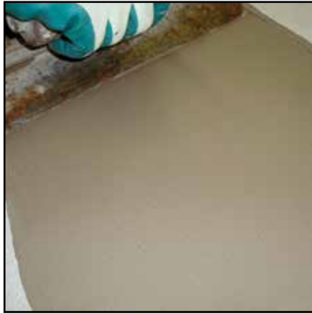
PRO PATCH™ used over concrete
