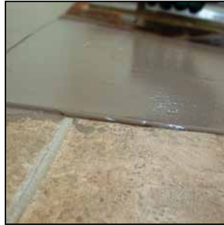
PRO PATCH™ mixed with PRO PATCH LIQUID™ used over non-cushioned vinyl sheet goods as an embossing leveler
