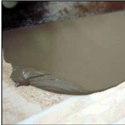
PRO PATCH SUPREME™ used as an embossing leveler over existing ceramic tile
