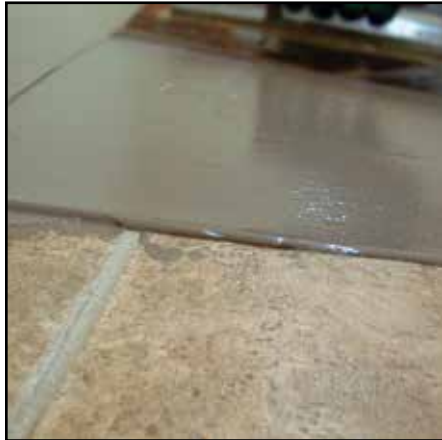
PRO PATCH™ mixed with PRO PATCH LIQUID™ used over non-cushioned vinyl sheet goods as an embossing leveler
